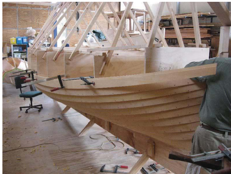
Figure 16: Clinker Construction Source: Woodwork Forums
