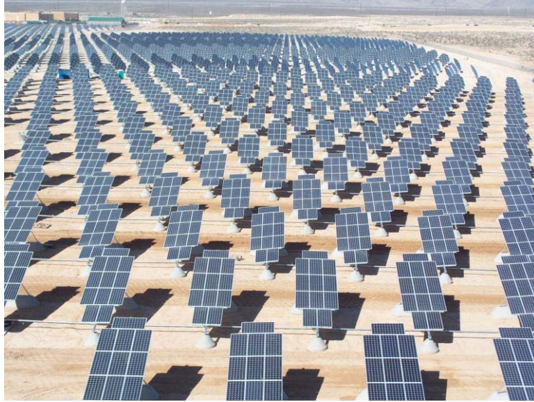
Figure 7: 14-MW Solar Array at Nellis Air Force Base Source: http://www.nellis.af.mil/nellissolararray.asp
